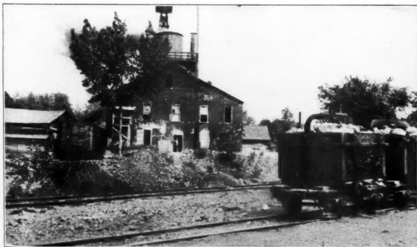
Boxes Loaded With Stone on Small Flat Cars Which Have Come from the Quarry
